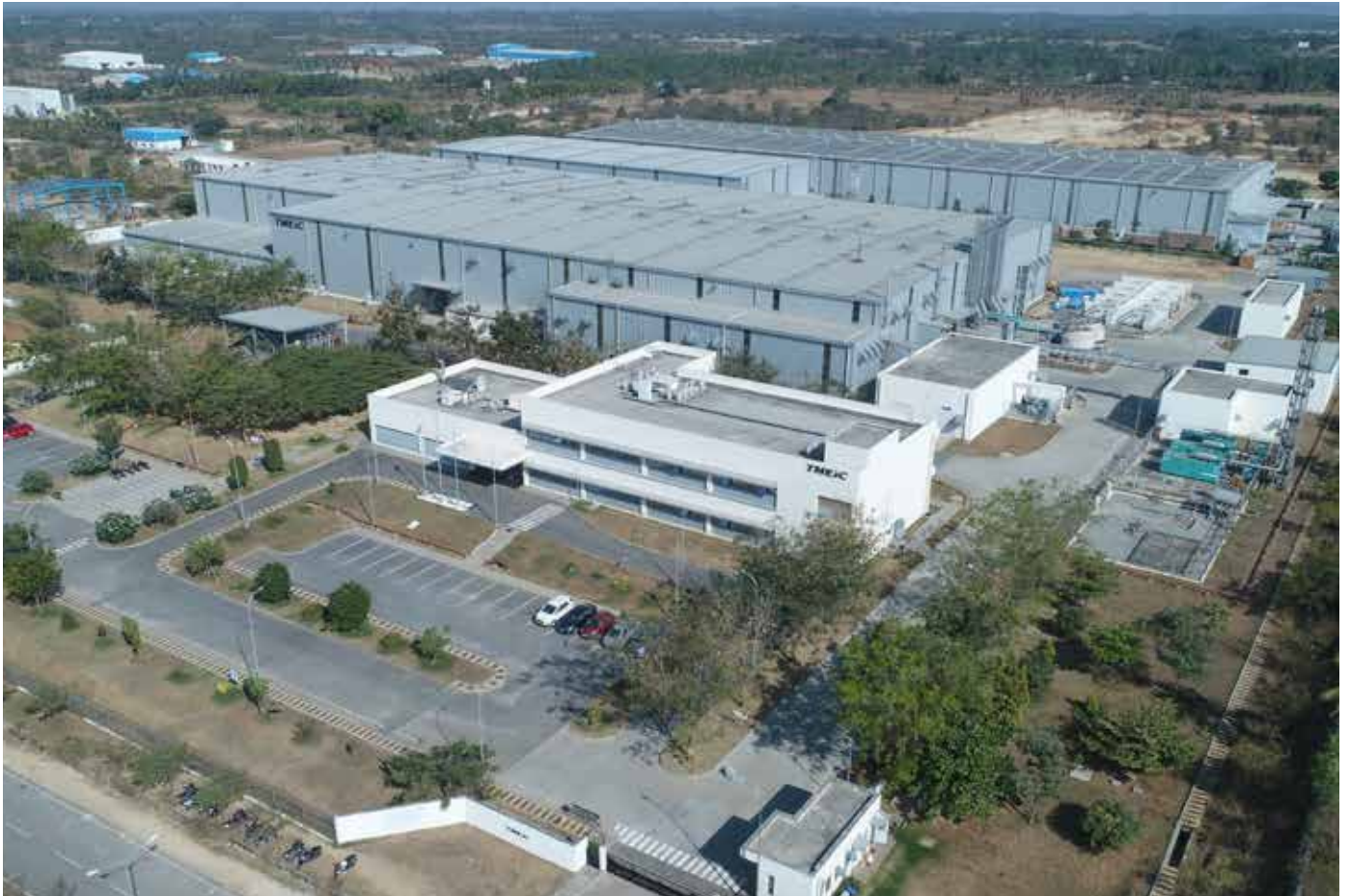
▲ Rotating Machine Factory & Power Electronics Factory (Tumakuru, Near Bengaluru)
